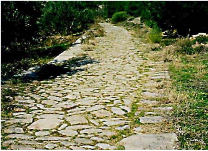
The Via Egnatia – The Egnatian Way was a road built by the Romans. It was well paved, and gently graded, allowing easy travel between Rome and Byzantium. Thessalonica was a major city on this road.
